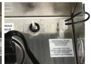
2. Unplug photocell plug from transformer.
