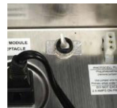
2. Unplug photocell plug from transformer.
