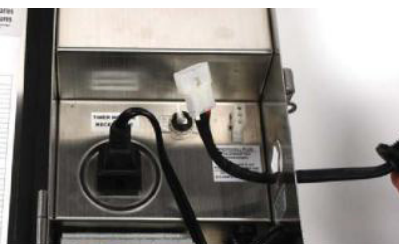
3. Insert the wire and connector of photocell through hole in side of transformer. Place nut around wire and screw onto photocell, holding unit in position.
