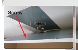
8. Lift panel onto remaining hooks on Surface Mounting Bracket while aligning to remaining slots on panel. Slide panel the same direction as step 4 until the panel locks into the second notch. (Fig. 8-1 & 8-2)
